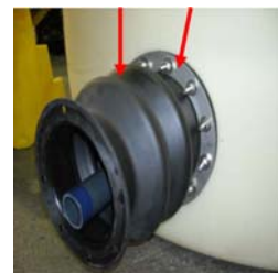
Install bellows and SS Back Rings
